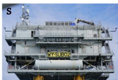
Figure 1 WOW02 OSS sides with their identifiable features. N- North face, identifiable as one of the larger sides with a crane at the top and no tank. E- East face, mooring ladders on yellow structural supports and stairs going up the left side. S- South face, large side with a storage tank at the bottom. W- West face with satellite tower on top and stairs up the right side.
