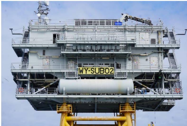
Figure 2: Full, face-on aspect image of the south side of WOW02 OSS.
