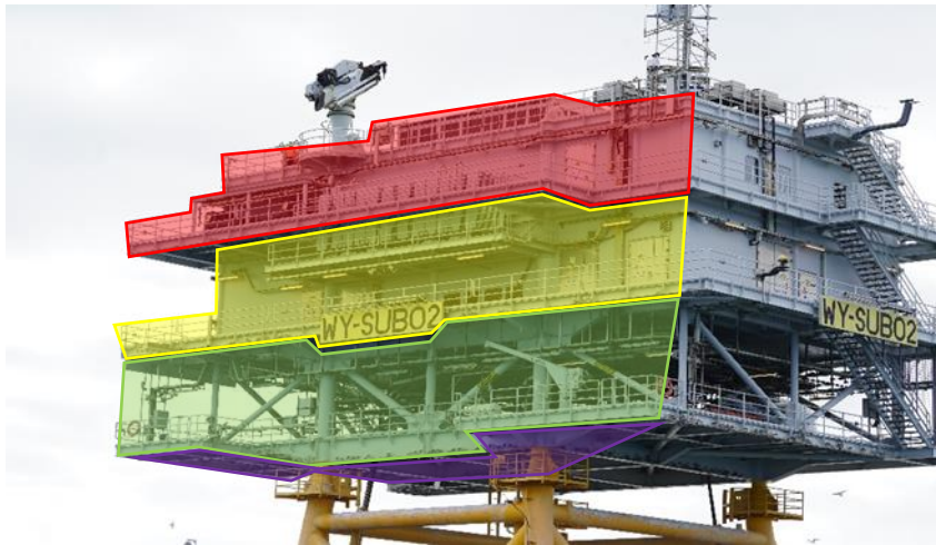
Figure 2d. Image of WOW02 OSS northside exemplifying how the substation was divided into layers: top (red), middle (yellow) and bottom (green) layers. The underside (purple) was categorised as a side.
