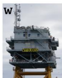
Figure 1 WOW02 OSS sides with their identifiable features. N- North face, identifiable as one of the larger sides with a crane at the top and no tank. E- East face, mooring ladders on yellow structural supports and stairs going up the left side. S- South face, large side with a storage tank at the bottom. W- West face with satellite tower on top and stairs up the right side.
